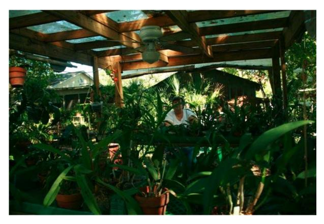
Bob has been busy creating different homes for their orchids. He has built a covered shade structure using  $4 \times 4$ 's in the corners with  $2 \times 8$  ceiling joists and stringers. There is a ceiling fan to keep air moving. There is corrugated plastic on the top of the structure to prevent waterlogging the orchids during tropical storms and hurricanes.
