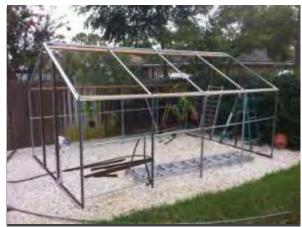
The rigid-frame structure has vertical sidewalls and rafters for a clear-span construction
