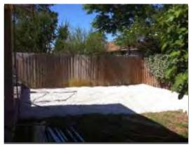
remove. I would recommend going at least three feet outside of the actual area where the greenhouse will be placed to ensure that no vegetation will grow into the structure itself. After tilling the ground and removing the vegetation, you need to level out the ground as best a possible.
